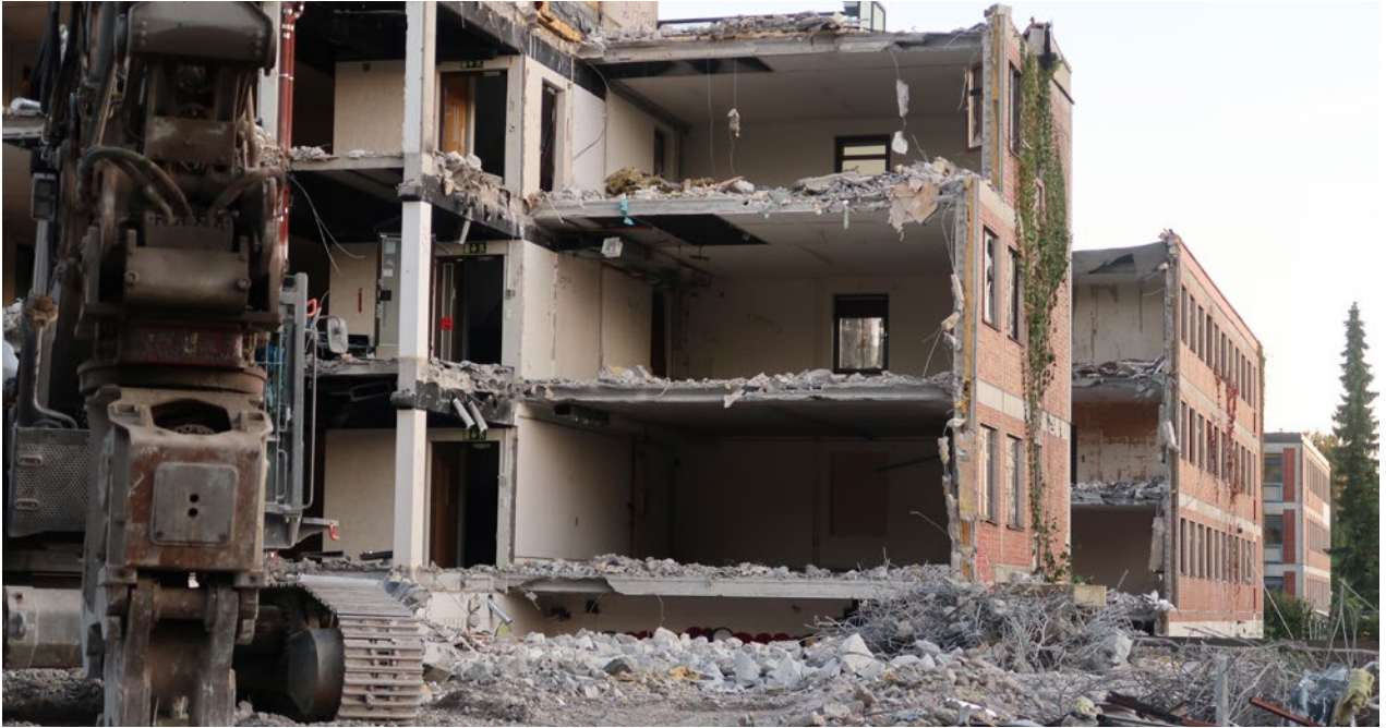
Three office buildings being demolished, Helsinki, Finland, 2020. Photographer: © Harri Hakaste
